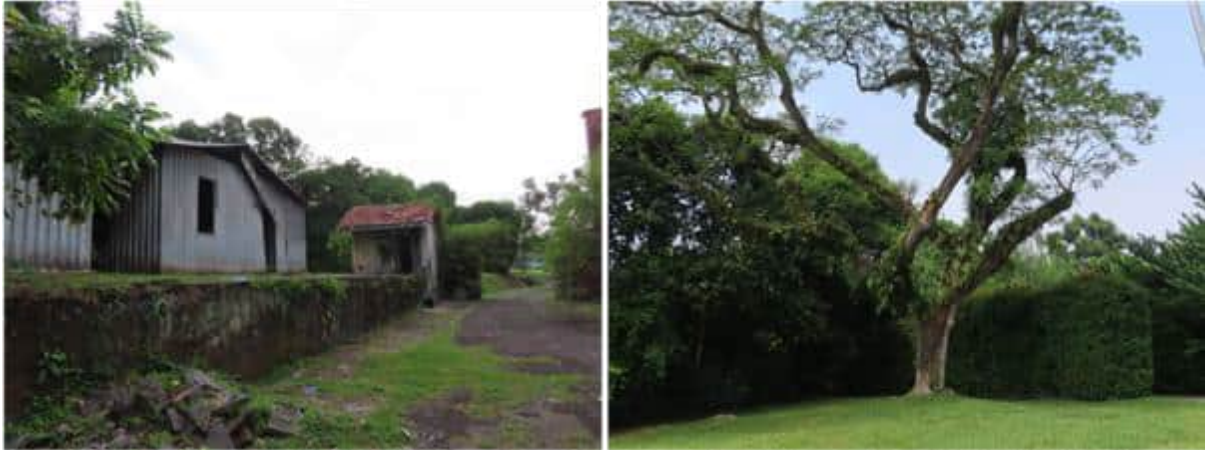
Figure 7-28 Urban vegetation and abandoned buildings at 700 Dunearn Road in Site E
