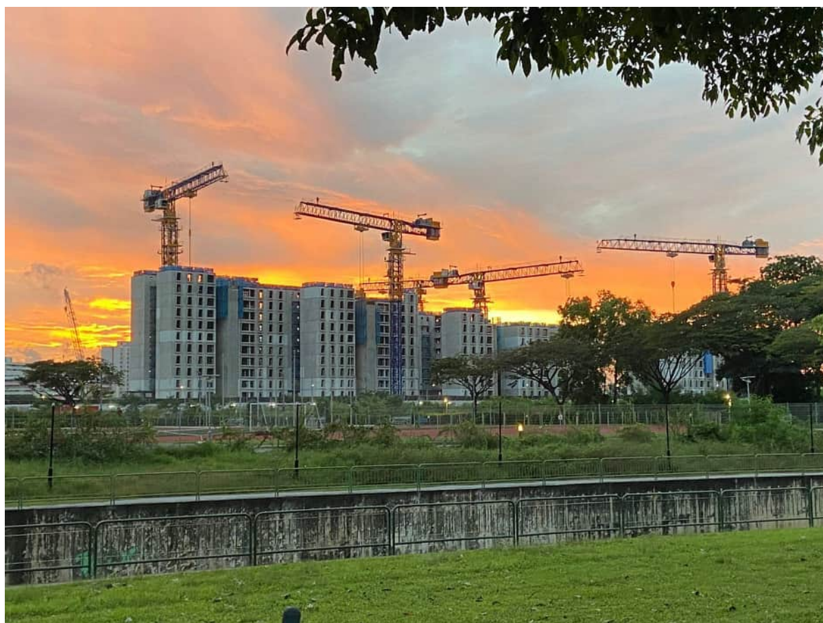
Figure 3-7 An example of superstructure construction works in Singapore (AECOM ©)
