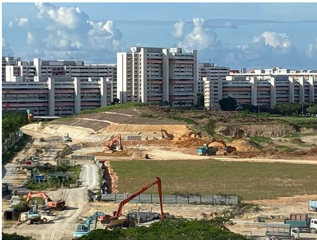
Figure 3-6 An example of site levelling at construction worksite in Singapore (AECOM©)
